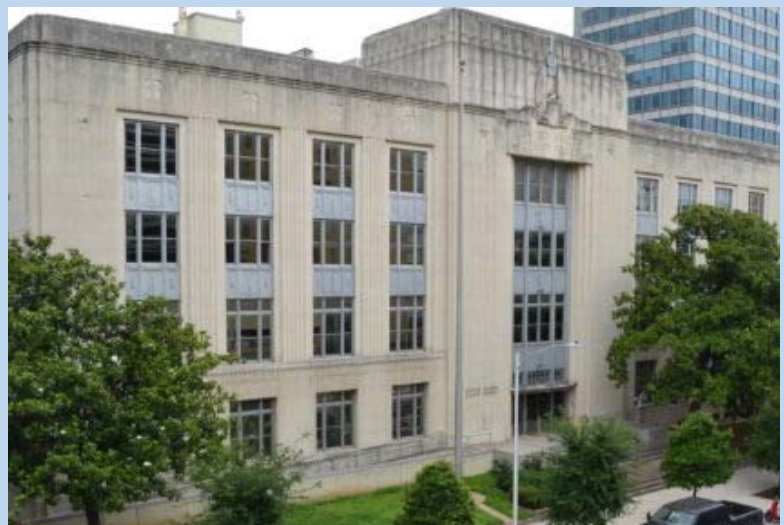
Historic Federal Courthouse
